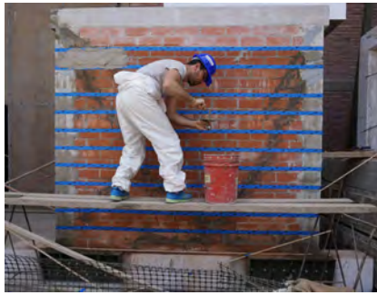
(a) First layer of mortar
