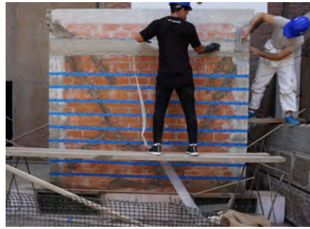
(b) Placement of steel fiber mesh
