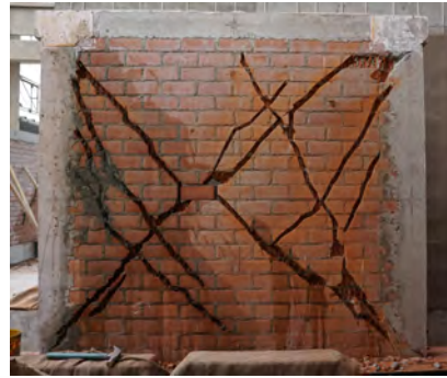
(b) Filling of openings
