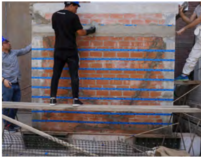
(c) Second layer of mortar
