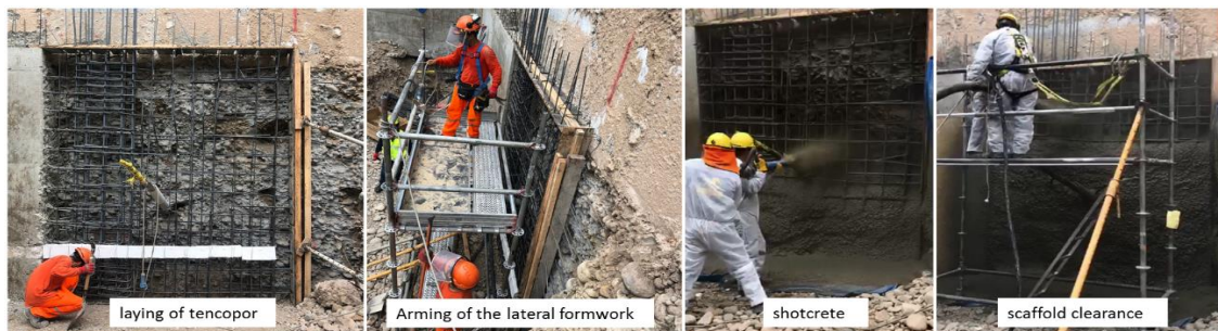
Figure 8. Additional activities with the Shotcrete System
