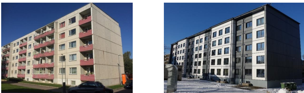
Figure 1. The building before (left) and after (right) renovation.
