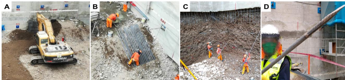
Figure 6. Improvements and innovations in basement construction.
