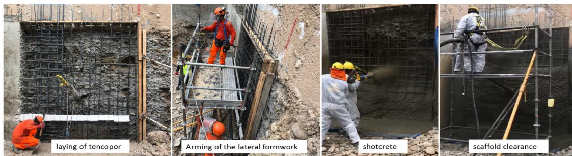
Figure 8. Additional activities with the Shotcrete System
