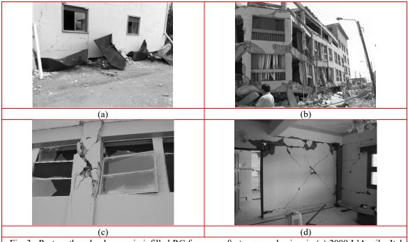
Fig. 3 Post-earthquake damage in infilled RC frames: soft-storey mechanism in (a) 2009 L'Aquila, Italy and (b) 2007 Pisco, Peru earthquakes; (c) short column effect in 2007 Pisco, Peru earthquake; (d) diagonal cracking at infill panels in 2001 Bhuj, India earthquake (Patel and Pindoria 2001).
