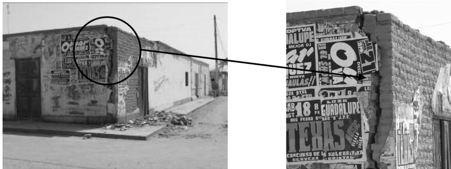
**Figure 2.** Vertical cracks at the corners of connecting adobe walls.
