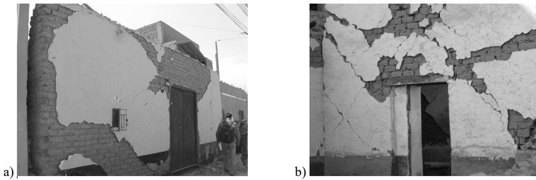
**Figure 8.** Failure of walls due to in-plane forces (see Table 2): (a) demand < LS4, (b) demand > LS4.
