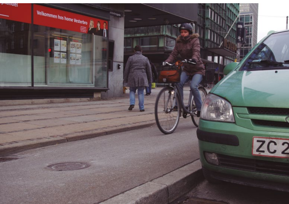
Traditional Copenhagen cycle track, showing the two kerbs which separate cyclists from both pedestrians and cars.
