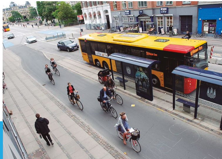
Approach road Nørrebrogade after rebuilding - note how wide the pavement and cycle track are.
