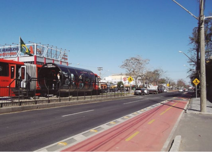
Figures 2 and 3. The municipality is remodeling its BRT corridors, and is implementing bike lanes along some of them, and installing bike racks near by the so called tube stations.
