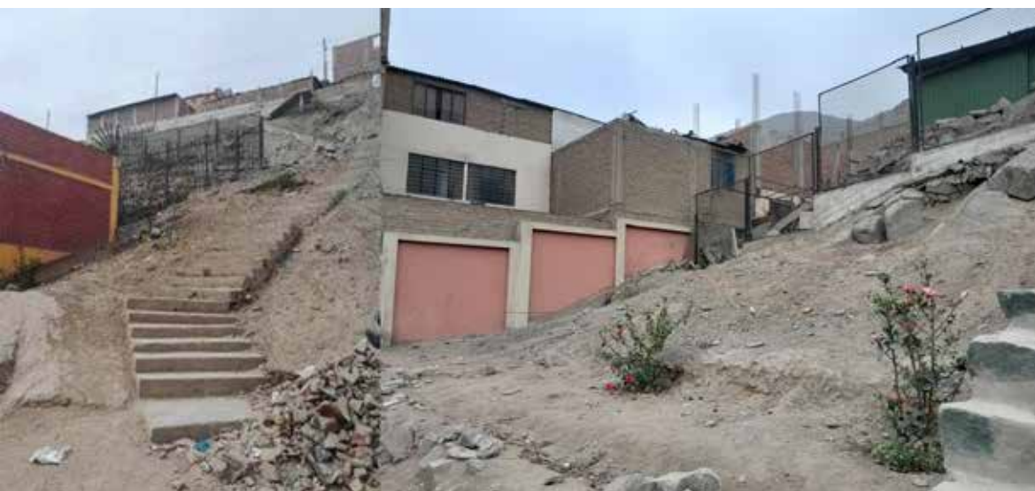
Perimeter fence wall at Okinawa Educational Institution
