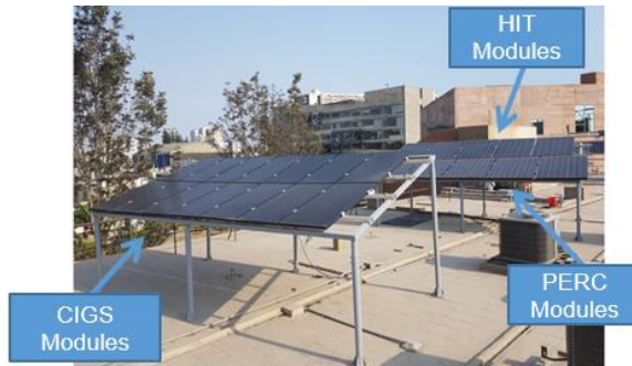
Figure 1. Installation of three different technologies at Physics section, PUCP, Lima, Peru.
