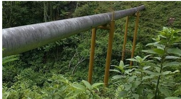
Figure 4. A view of the oil pipeline under study.
